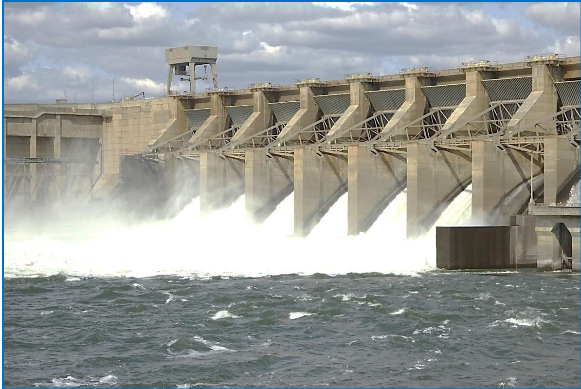
Ice Harbor Dam Tailrace, Lower Snake River (2023)
